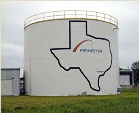
Arkema plant in Crosby, Texas
