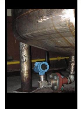
"If I see a problem in some part of our process, it is fairly simple for me to take a pressure transmitter and move it elsewhere. I can often determine what's going on in just five minutes, address the issue and quickly return the transmitter to its original application. The flexibility of Emerson's self-organizing wireless technology makes it much easier to troubleshoot problems as well as evaluate new applications."
